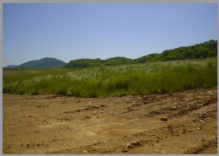
Sevier Solid Waste Inc. used compost as a final layer to cap an old landfill. Compost used with dirt to make a 70/30 soil blend to cover. Hydroseed was also applied with the soil mixture. After just one season, this is the grassy field that remains of the landfill.
