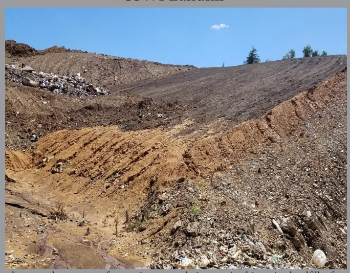
Sevier Solid Waste Inc also uses the compost for erosion control. As seen in this active landfill, after a heavy rain there was serious runoff. The dark layer of dirt is our compost. Applied at about 2inches depth over this slope, it absorbed the majority of the rainfall. At the bottom of the slope, you can see evidence of erosion in the rivets in the dirt. This is a good example of how our compost can control erosion as opposed to the natural dirt of the area.
