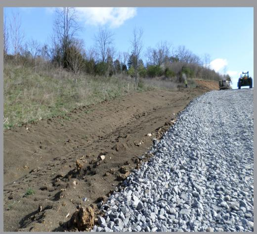
Sevier Solid Waste Inc. used compost on a new entrance to a working landfill. We used the compost on the shoulder to improve vegetation and for erosion control down the hill leading to the road. Compost was applied with a small blower truck on the gentle slopes of the side banks and along the shoulder of the new gravel road.
