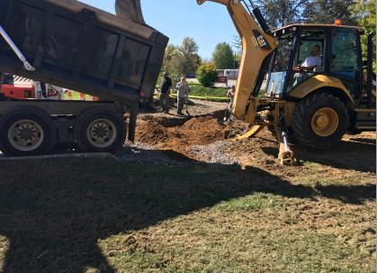
Here is the Sevierville Public Works rain garden under construction. They added compost to the existing sublayers of soil. The compost was then able to absorb and hold water that was previously flooding the area.
